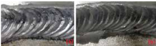
Figure 2. The welding joints of S-1(a) and S-2(b)
