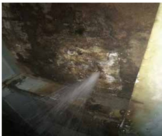
Figure 5. Granulated Inba Chimney Floor Drilling
